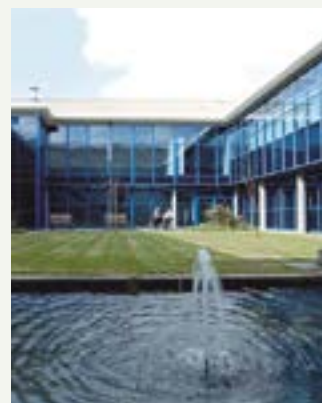
NHS Canford house clinic, Bournemouth, UK. VRF
