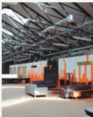
Zalando's solution for its warehouse office conversion at Grand Canal Quay, Dublin. ECOi
