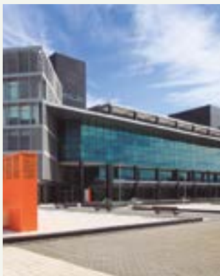
Andalucia Technology Park. Offices of high energetic efficiency. Spain. ECOi
