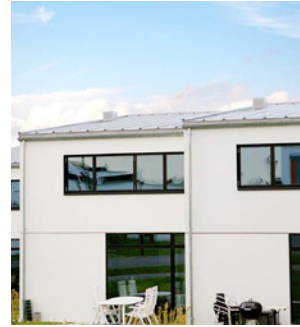
75 low-energy-consumption houses in Hasselager (Denmark)
