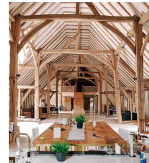
17th century barn renovation with floor heating in Essex (UK)
