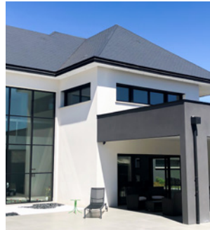
610m² house with underfloor heating and DHW in Saint-Prest (France)
