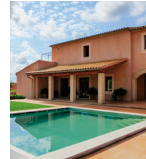
Premium passive refurbishment villa "Projecto Tierra" in Lluçmajor, Mallorca (Spain)
