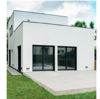
New passive house in Sant Cugat del Vallès (Spain)
