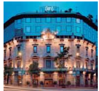
Hotel refurbishment. Hotel Claris 5 * Barcelona, Spain. ECOi
