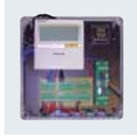
Air Handling unit kit connected to the ECOi and PACi system.
