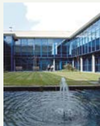
NHS Canford house clinic, Bournemouth, UK. VRF
