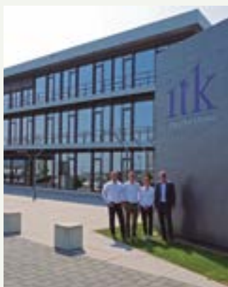
ITK Engineering GmbH. An innovative office building located in Germany. ECOi - PACi
