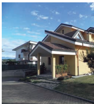
Duplex in Boves, CN. Italy. AQUAREA
