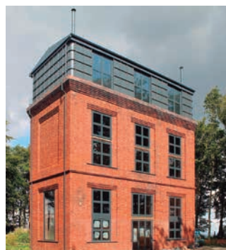
An water tower has been converted into a stunning family home. Yorkshire, UK. AQUAREA
