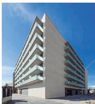
A new building, housing 84 apartments in Cornella de Llobregat, Barcelona. AQUAREA
