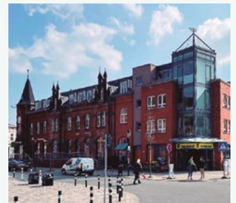
The EDEKA store in Germany, the first supermarket providing the maintenance-free nanoe™ X technology for better indoor air quality. Germany. ECOi and nanoe™ X
