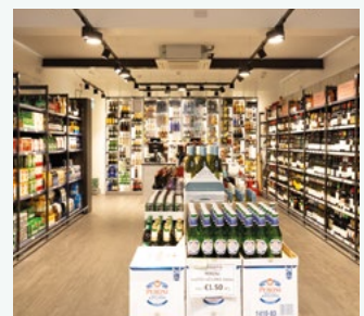
Nolan's supermarket in Ireland installs the first Panasonic CO 2 condensing units - CR Series for showcases. Ireland. Refrigeration
