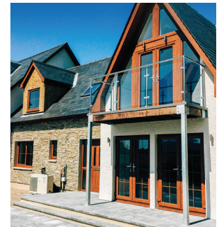
Tower Ridge Courtyard i Skottland (Storbritannia)
