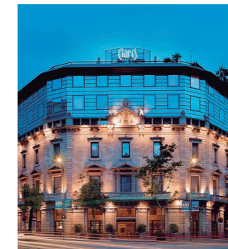
Hotel refurbishment. The heat recovery system is ideal for a hotel of this category. Hotel Claris 5*. Barcelona, Spain. ECOi
