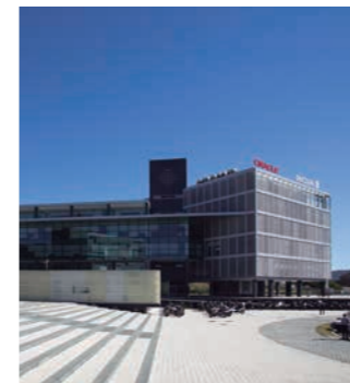
Andalucia Technology Park. Málaga, Spain. ECOi
