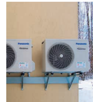
PKEA for Server Room. Munich Municipal Hospital. Germany. PACi
