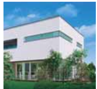
Smart House. Ariake, Tokyo. HVAC and the combination of solar power generation, fuel cells and storage batteries.
