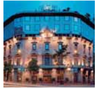
Hotel refurbishment. Hotel Claris 5 * Barcelona, Spain. ECOi
