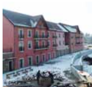
Montcenis Nursing Home. Over 6100 m 2 and 85 rooms. Saône et Loire, France. ECO-G
