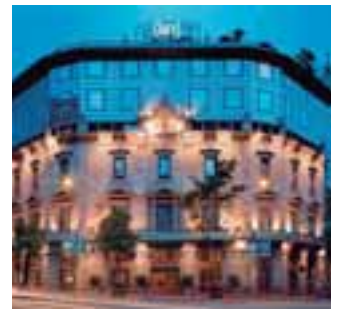
Hotel refurbishment. Hotel Claris 5 * Barcelona, Spain. ECOi
