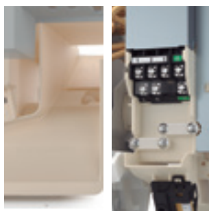
Bigger working space for wiring connection.
