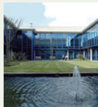
NHS Canford house clinic, Bournemouth, UK. VRF
