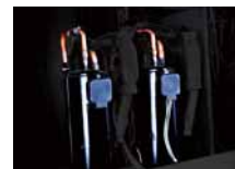
Multiple large-capacity all inverter compressors (more than 14 HP).
