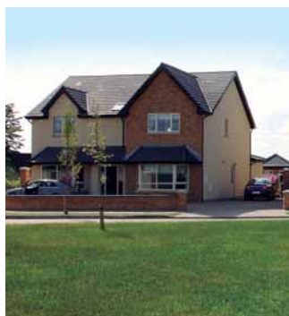
21 of the 5-6 bedroom luxury homes in Straffan Co.Kildare, Ireland. Aquarea
