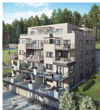
New condominium. Bergås Terrasse complex. Drammen, Norway. ECOi / Aquarea
