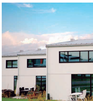
Brabrand Boligforening has constructed 75 low-energy houses in Hasselager near Århus Denmark. Aquarea
