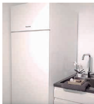
Five new terraced houses in Herlev. Herlev, Denmark. Aquarea
