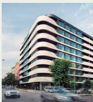
Bulgaria's stand-out residential building with efficient HVAC solution. Aquarea
