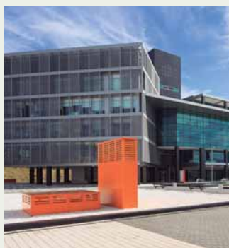
Andalusia Technology Park. Offices of high energetic efficiency. Spain. ECOi
