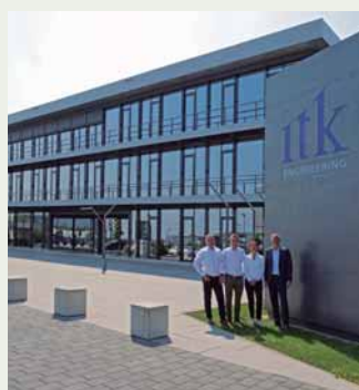
ITK Engineering GmbH. An innovative office building located in Germany. ECOi - PACi
