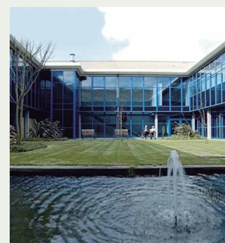
NHS Canford house clinic, Bournemouth, UK. VRF
