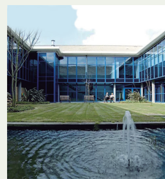
NHS Canford house clinic, Bournemouth, UK. VRF
